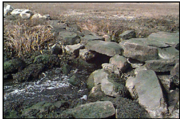
Old stone culvert at Restriction DA15
