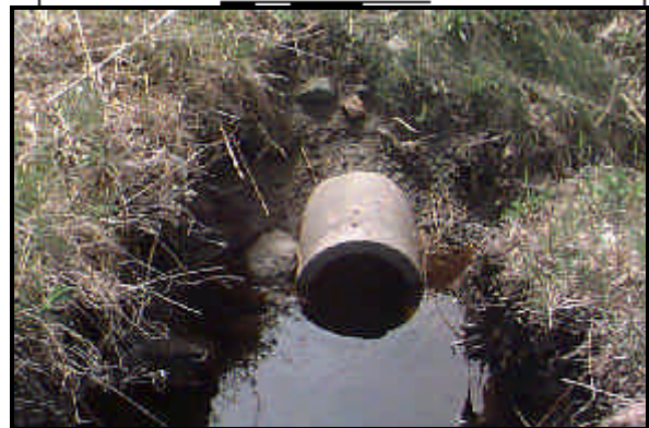
Culvert under Fir Street, upstream side
