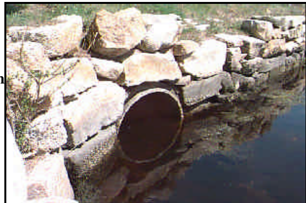
Upstream side of tidal restriction MT03
