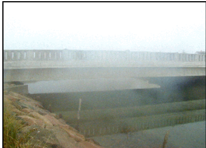
New Bridge at Old Silver Beach (FA23).
