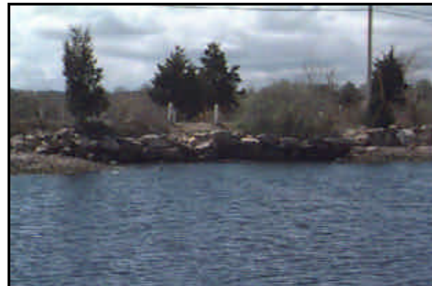
Downstream side of tidal restriction MT03
