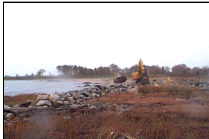
Removal of restriction MN22 (a stone wall across a salt marsh) during 1999.
