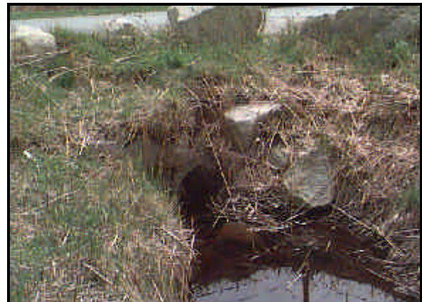
Culvert under Fir Street, downstream side
