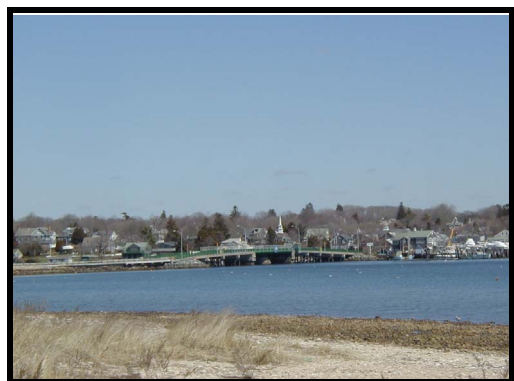
View of bridge and road
