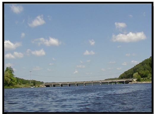
View of Hix Bridge, looking North
