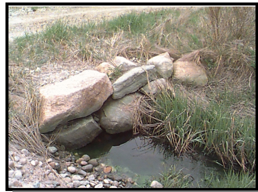
South side of culvert
