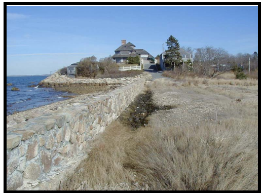
View of rock wall
