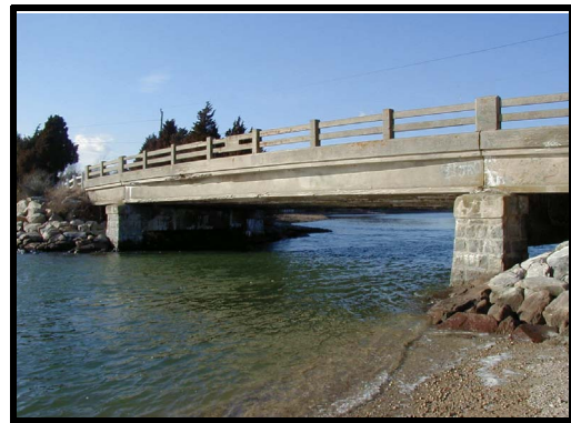
South side of bridge looking upstream
