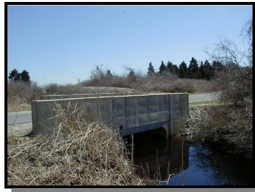
Culvert under road
