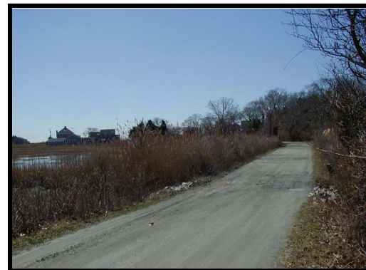
Gravel road passing over restriction DA06
