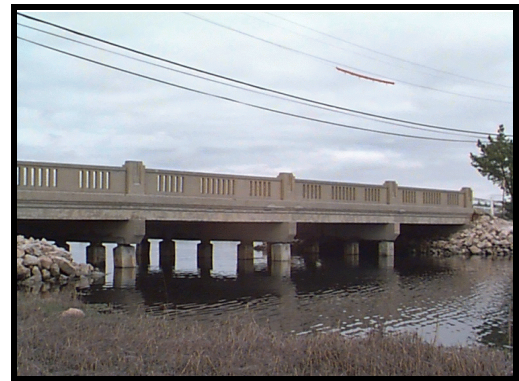
View of bridge
