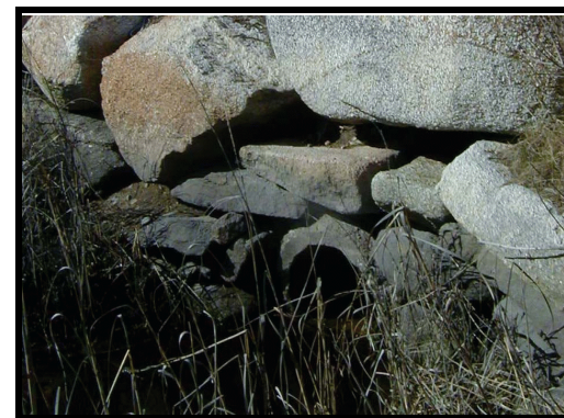
Upstream end of culvert
