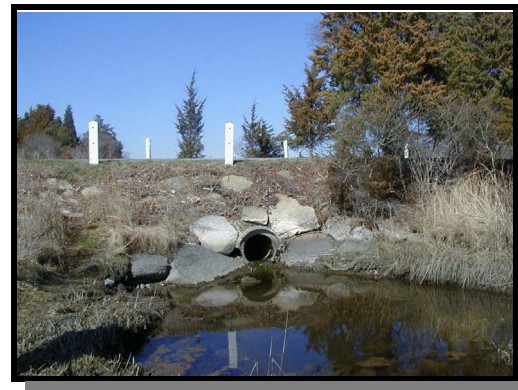
View of south side of Mattapoisett Neck Road
