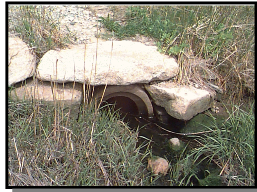
North side of culvert
