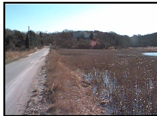
View of road
