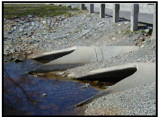
South end of culverts
