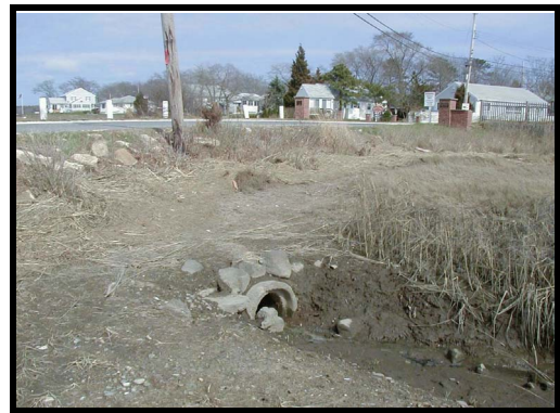
East end of pipe
