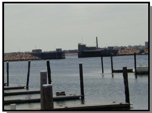
Opening in hurricane dike from the Fairhaven Shipyard & Marina
