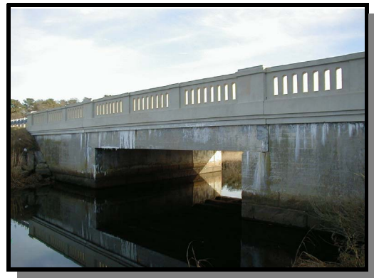
North side of bridge
