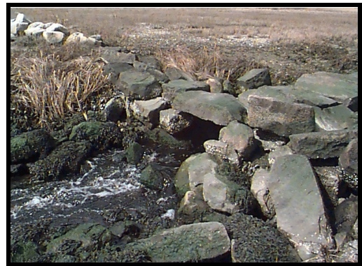
Old stone box culvert
