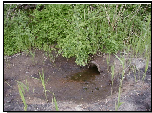
Mill Pond side of culvert
