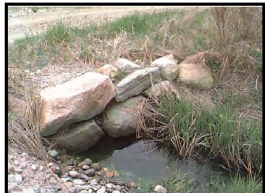
South side of culvert
