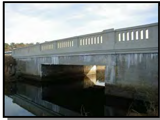
North side of bridge
