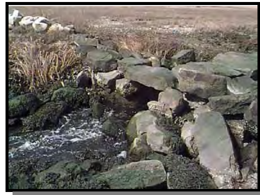
Old stone box culvert
