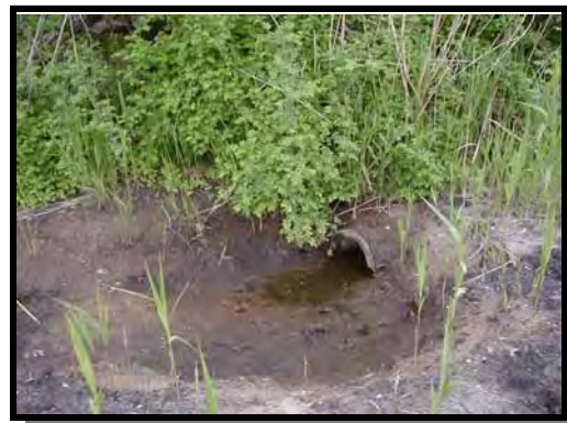
Mill Pond side of culvert
