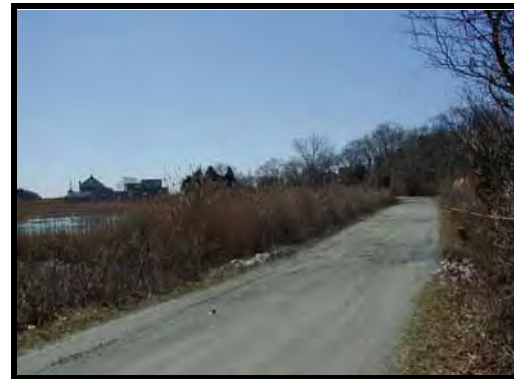
Gravel road passing over restriction DA06
