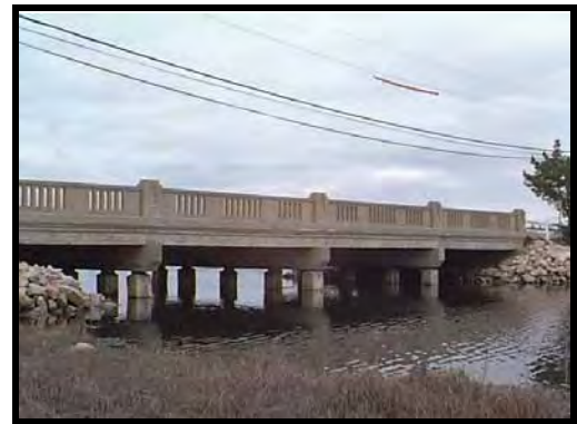
View of bridge
