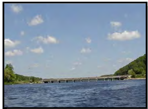
View of Hix Bridge, looking North
