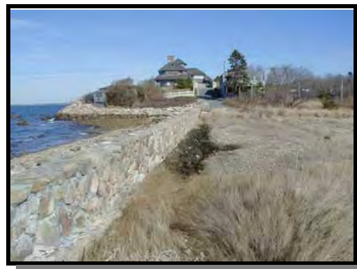
View of rock wall
