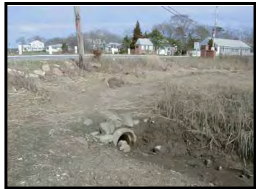
East end of pipe
