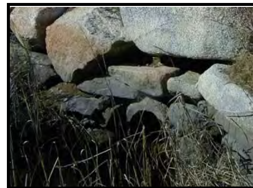
Upstream end of culvert
