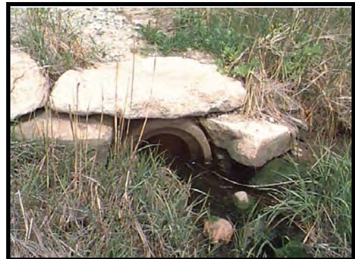
North side of culvert
