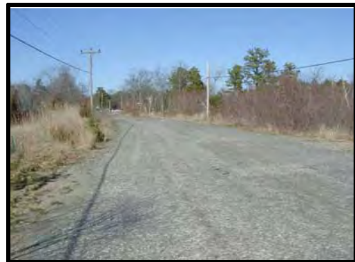
Old section of Route 6
