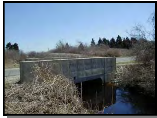
Culvert under road
