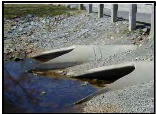
South end of culverts
