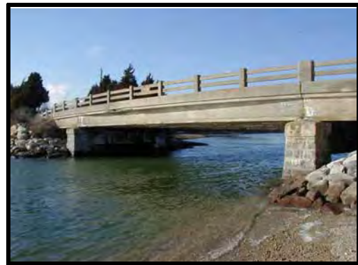
South side of bridge looking upstream
