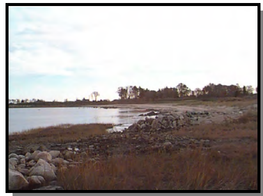
Section of wall that was removed
