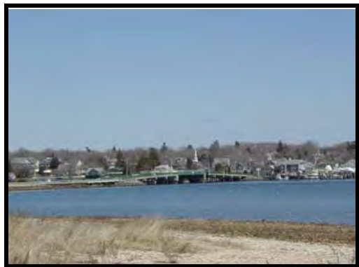
View of bridge and road
