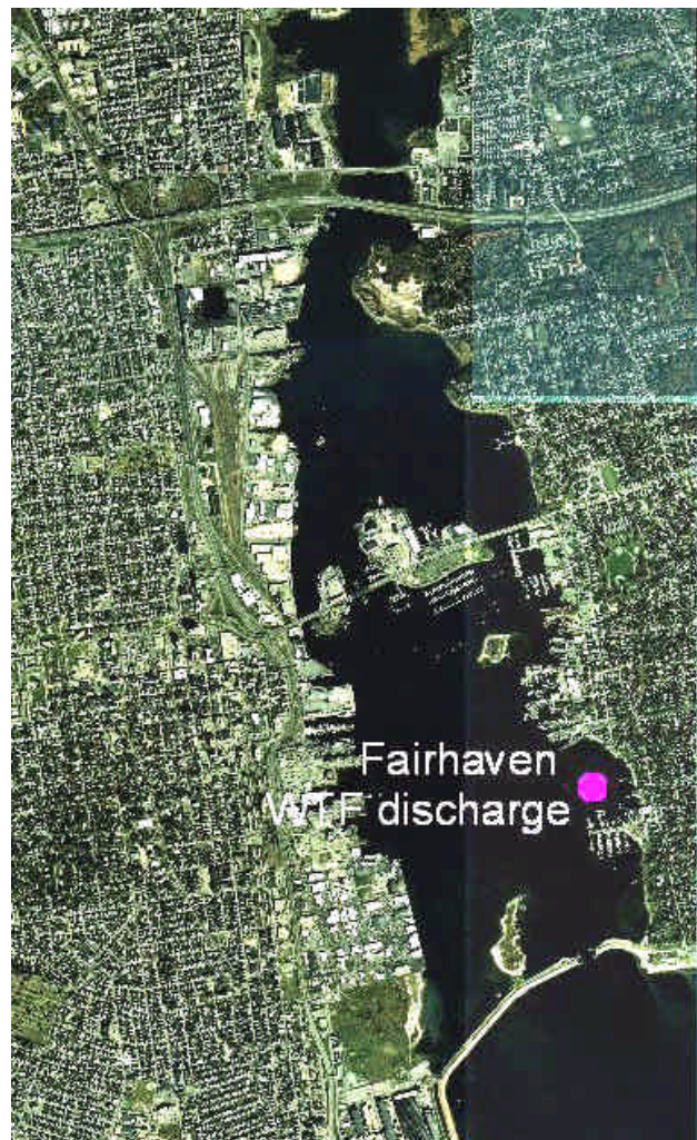
Figure 1. Aerial view, circa 1991, of central New Bedford Harbor, showing the approximate location of the outfall of the Fairhaven Wastewater Treatment Facility.
