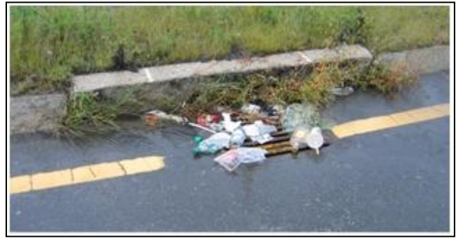
Figure 94. Litter accumulating on a storm drain grate.
