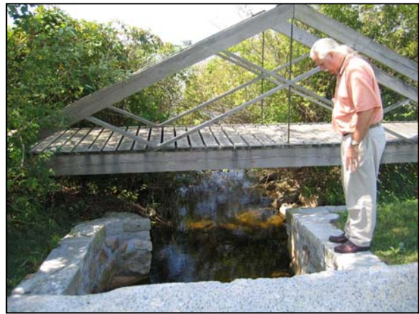
Figure 72. This water level control structure at Cockeast Pond Westport was modified to enhance herring passage.
