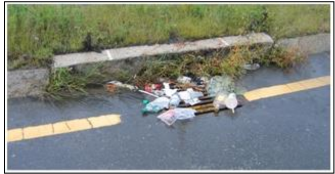
Figure 94. Litter accumulating on a storm drain grate.
