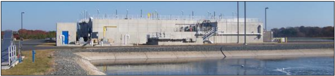
Figure 27. Town of Falmouth wastewater facility.
