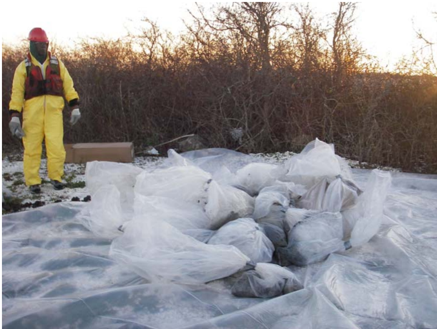
8. Remediation waste temporarily stored on-site in polyethylene bags.
