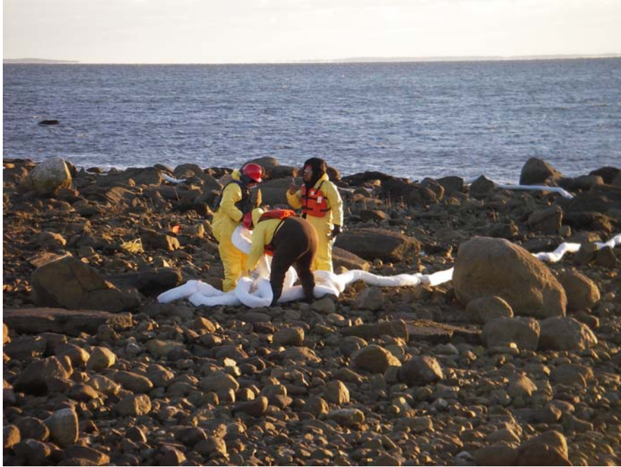
7. Oil absorbent boom installed along perimeter of the cleanup area.
