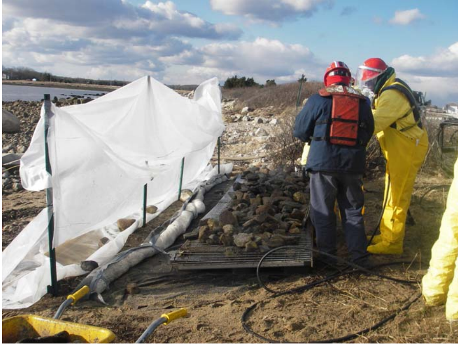
5. View of pressure washing containment area.
