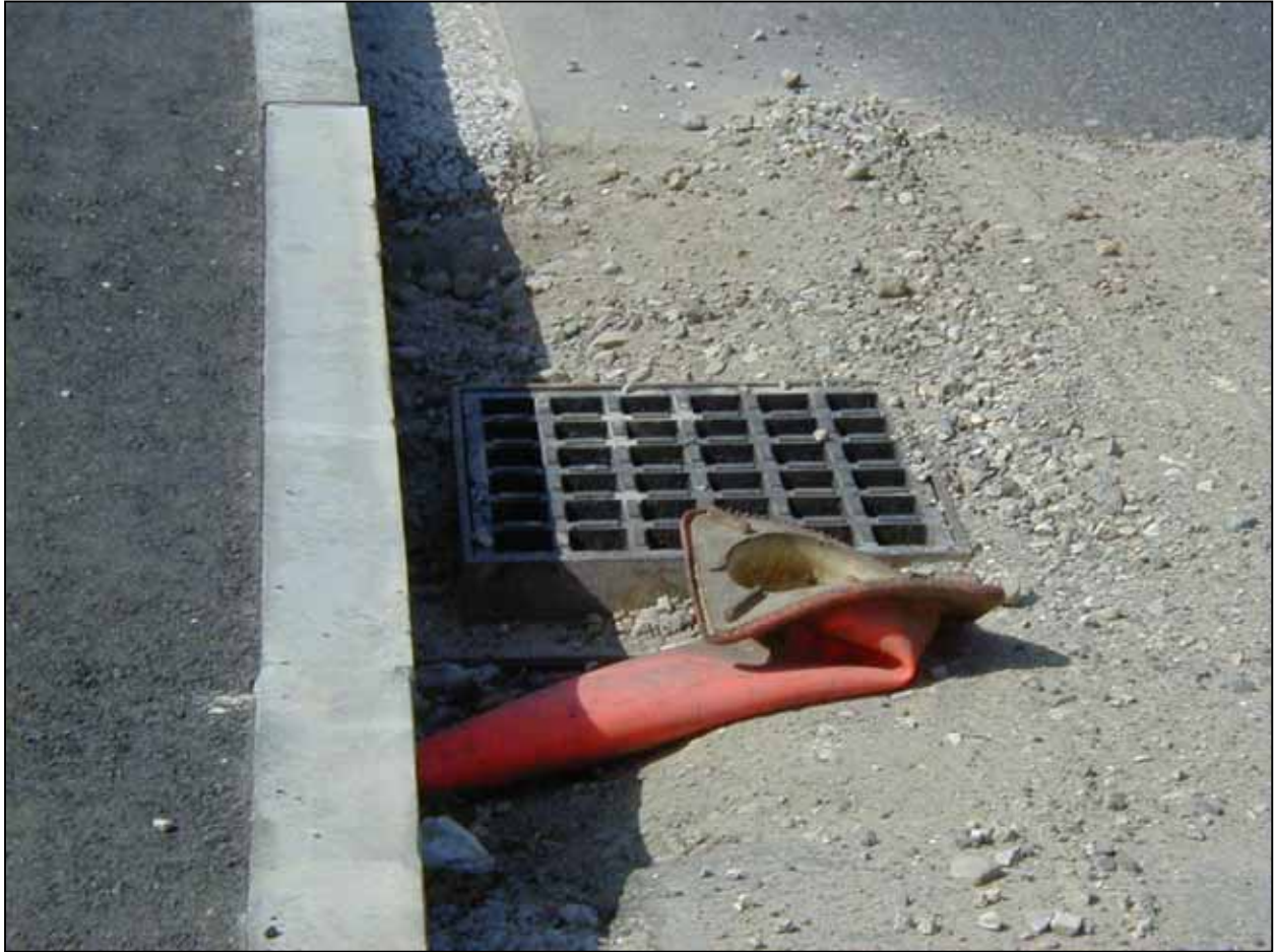
Figure 16. Photograph taken July 26, 2004 by the Buzzards Bay Project showing existing road conditions in the vicinity of the grates at the discharge points to the ponds.
