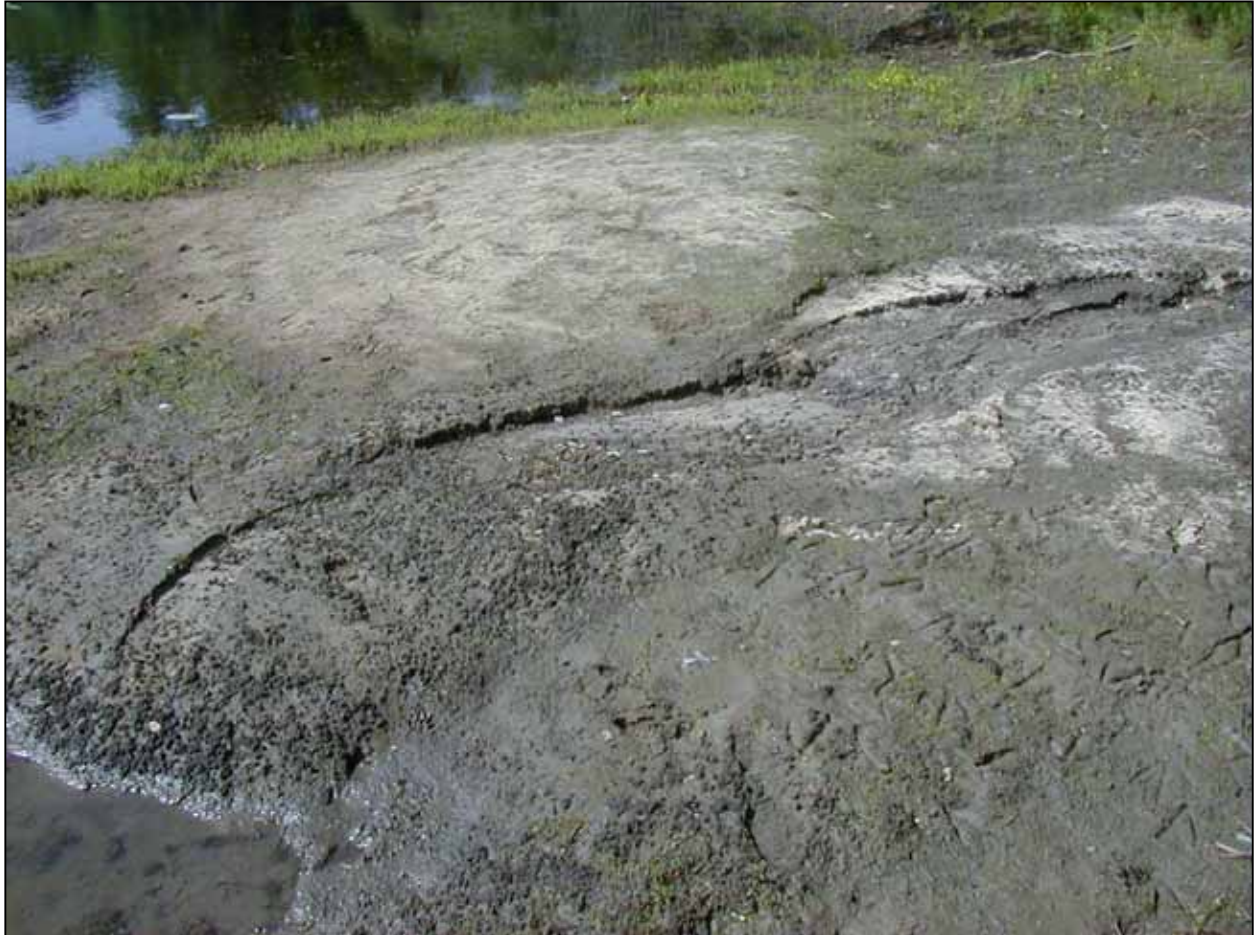
Figure 14. Photograph taken July 26, 2004 by the Buzzards Bay Project during low water pond conditions at Sols Pond along Gifford Street showing a sediment outwash “delta” near one of three observed discharge pipes from the road.
