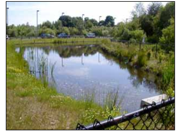
A stormwater detention pond serving a Falmouth shopping area parking lot.
