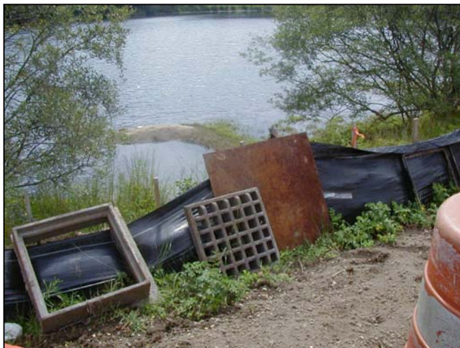
Fig. 1. Steel plate used to cover catchbasins near Sols Pond.
