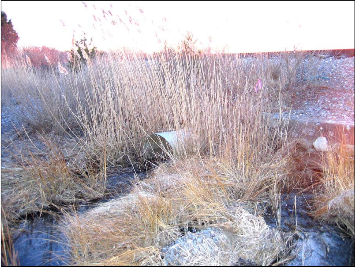
Figure 7. Photo of the landward side of the tracks at tidal restrictions FA28A and FA28 in Great Sippewisset Marsh. The old stone box culvert (right) is filled with boulders and track ballast stone. The metal pipe (FA28A left), probably installed after Hurricane Bob damage, was improperly sized and not at the correct elevation. A 400 square foot wetlands fill caused by a debris field of ballast from the Hurricane Bob washout begins to the left in this photo.
