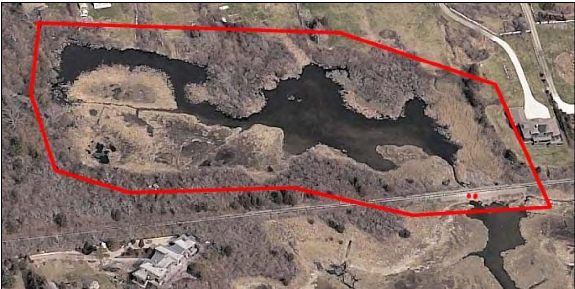
Figure 4. Oblique aerial photograph of restriction pipes FA28 and FA28A.
