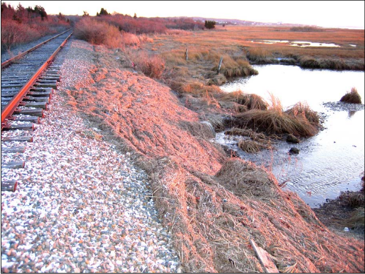
Figure 9. Spring high and storm surge wrack lines on the westward face of the tracks at restriction FA 28 and FA28A (pipe just visible center). The railway bed is at its lowest elevation in this location, and appears to be eroding on the seaward face.
