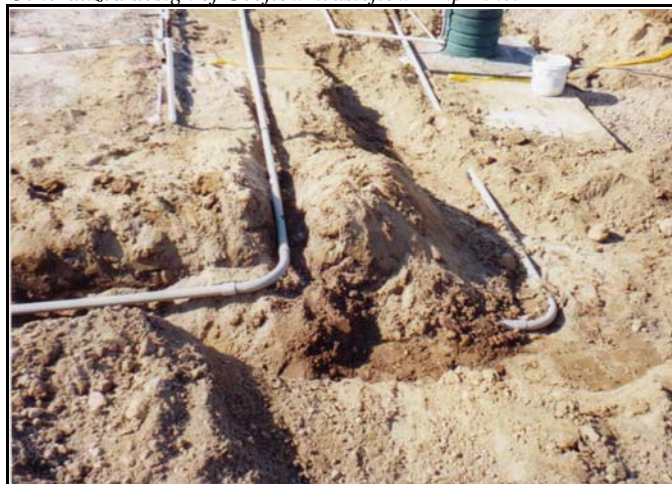
Drip Lines shown during installation.
