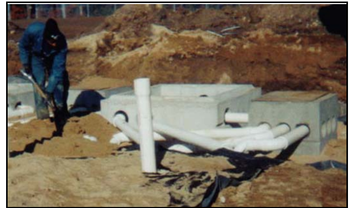
During installation, interplay box shown at right.
