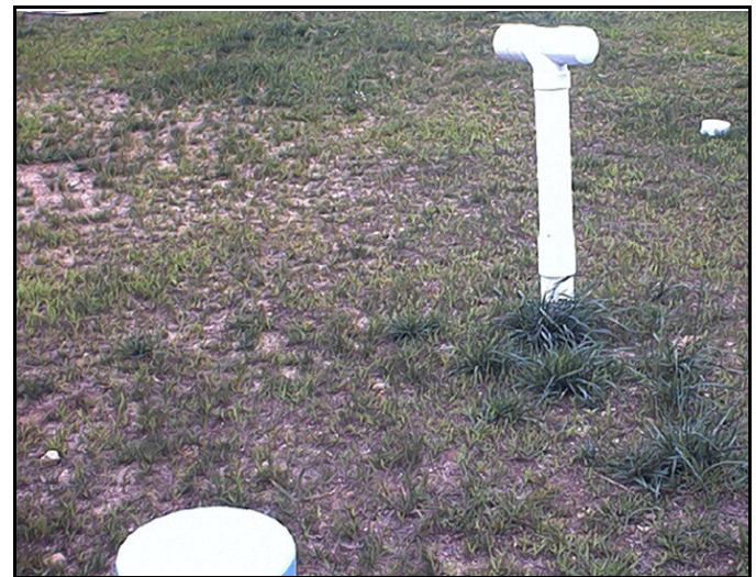
Final above ground view: aeration pipe and monitoring ports.
