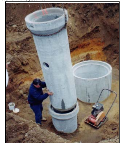
Installation of Amphidrome Unit.
