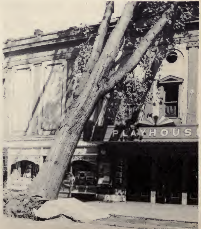
A mighty elm leaned against the top of the Playhouse Theater, uprooting yards of sidewalk as it fell, and battered down a chimney, showering tons of brick and plaster through the roof. Two men in the audience were injured.
