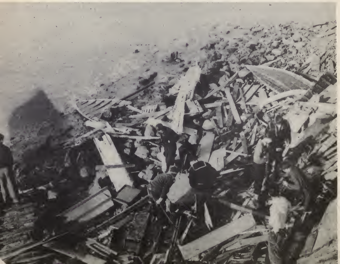
On the road to LYNN, an open-air "automobile" moving-picture theatre was blown apart, while in the city proper havoc was wreaked on houses and trees and telegraph poles.
