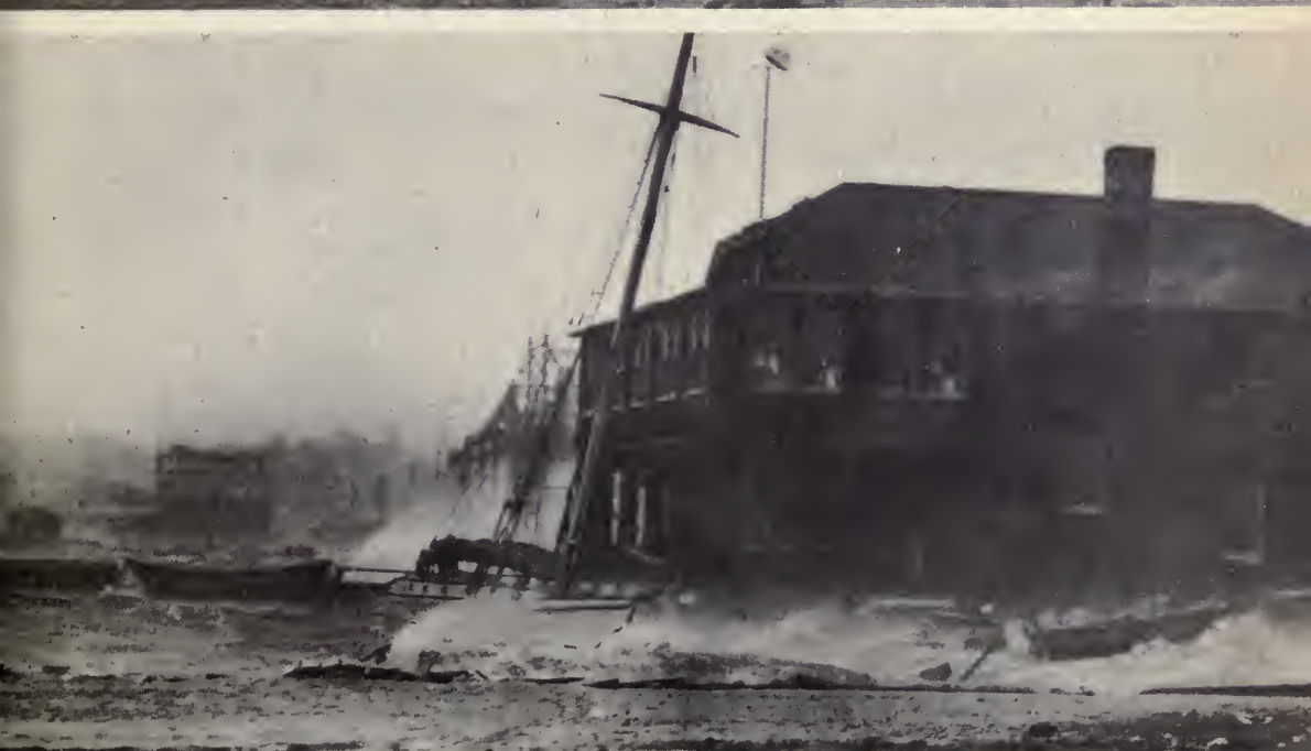
The New Bedford Yacht Club was plucked bodily from its foundation and scattered in broken wreckage on the surface of the New Bedford-Fairhaven bridge. This occurred 15 minutes after the photograph of the club was taken; members may be seen peering at the storm from windows. All escaped.
