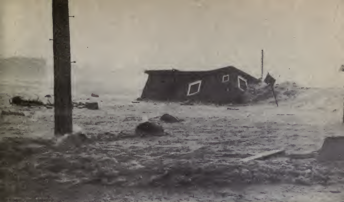
Cove Road , ordinarily a broad thoroughfare, became the graveyard of scores of small houses shortly after this picture was taken. The road was covered by 12 to 15 feet of water. The Kilburn Mill in the background was partially inundated.
