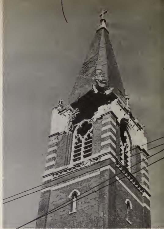
Northeast of Yantic, JEWETT CITY saw its imposing brick church put up a valiant fight against the hurricane. Twice the steeple appeared ready to go. A low-flying plane might have smashed that gaping hole in the belfry. The hole widened under terrific pressure. Miraculously, the steeple stayed aloft.
