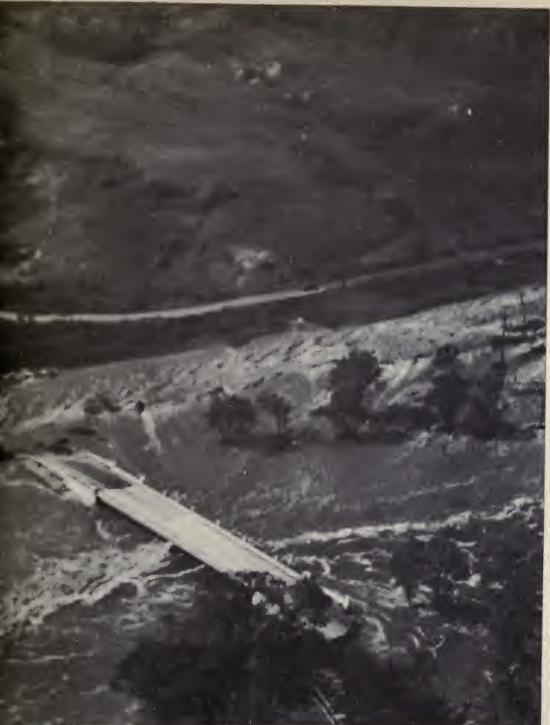
The Ware River rampaged through the Thorndike area. The 75-year-old covered bridge at Forest Lake, long a landmark, floated down stream and leaned against a lower bridge. The Church Street Bridge went out. At noon on Wednesday the 100-foot chimney of the No. 1 Thorndike Mill pitched into the water, which was nibbling away the building piece by piece. In the Three Rivers village bridges and roads collapsed; the center of town was flood-swept; 34 families lost everything they owned.
