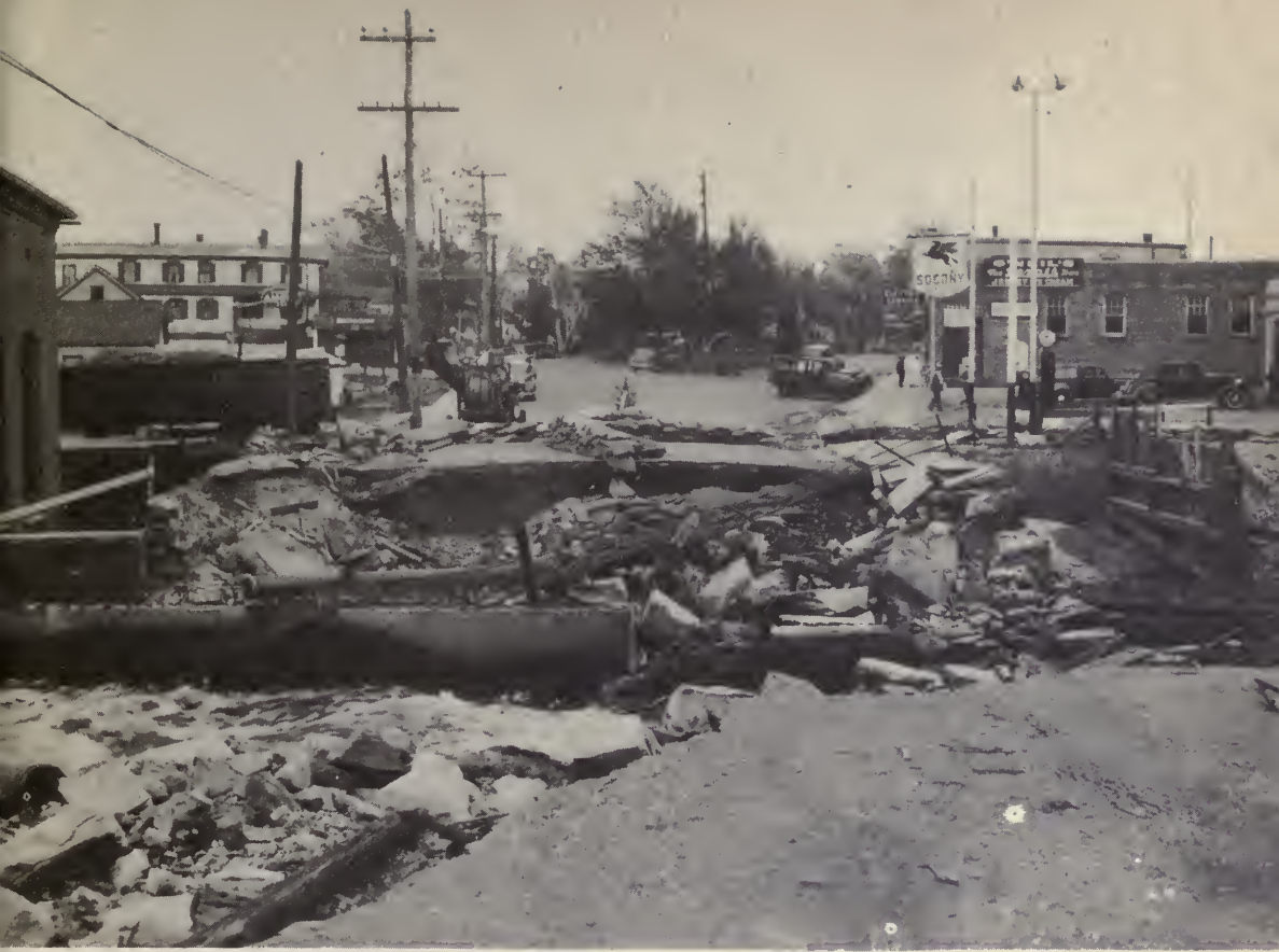
The bridge on Main Street in JAFFREY, on the southern shoulder of Grand Monadnock, is a jagged pile of asphalt and rocks. The shaded road from Jaffrey to Gilmore Lake is striped with fallen logs.
