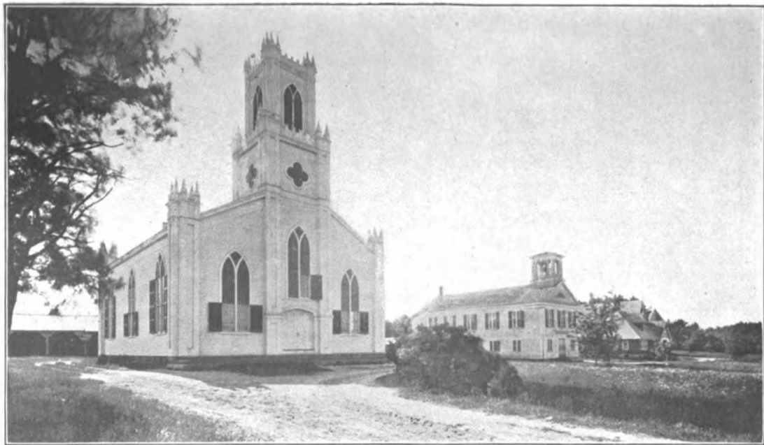
MEETING-HOUSE OF THE FIRST PARISH Showing the Academy and Town Hall Building, Rochester Center
