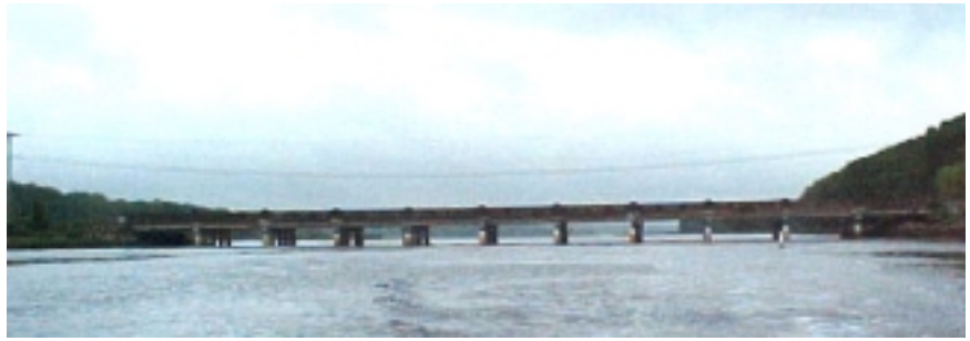
Figure 1. Hix Bridge today.
