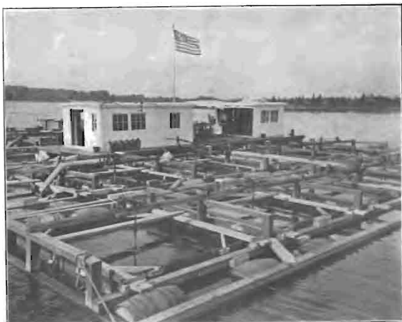
General view of plant from outer rear corner, starboard side. In foreground one car shows propeller shaft, and faint indication of propeller blades in water. The shaft coming through side of engine house passes into extension device seen just outside first shaft-hanger, then connects with longitudinal shafts. Location of rearing cars and alleys with barrels. (Reproduced by courtesy of Dr. A. D. Mead.)
