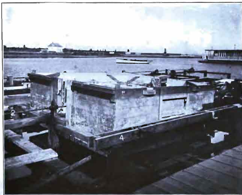
Rear of car raised and held up by portable windlass, showing slot in end of car, through which, when car is raised, longitudinal shaft runs (1); longitudinal shaft (2); side window of car (3); portable "horse" and windlass (4). (Reproduced by courtesy of Dr. A. D. Mead.)
