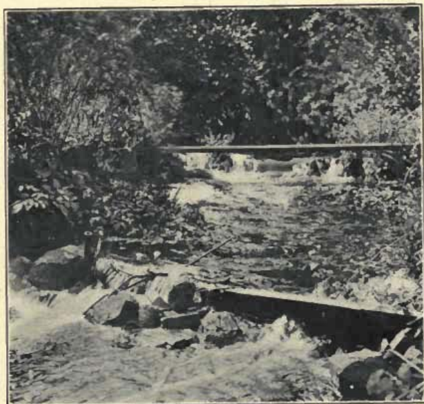
FIG. 8. — Obstructing material in Chebaeco Brook, Essex River.
