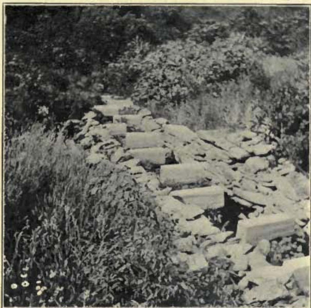
FIG. 11. — Stone fishway with concrete baffles, Nemasket River.
