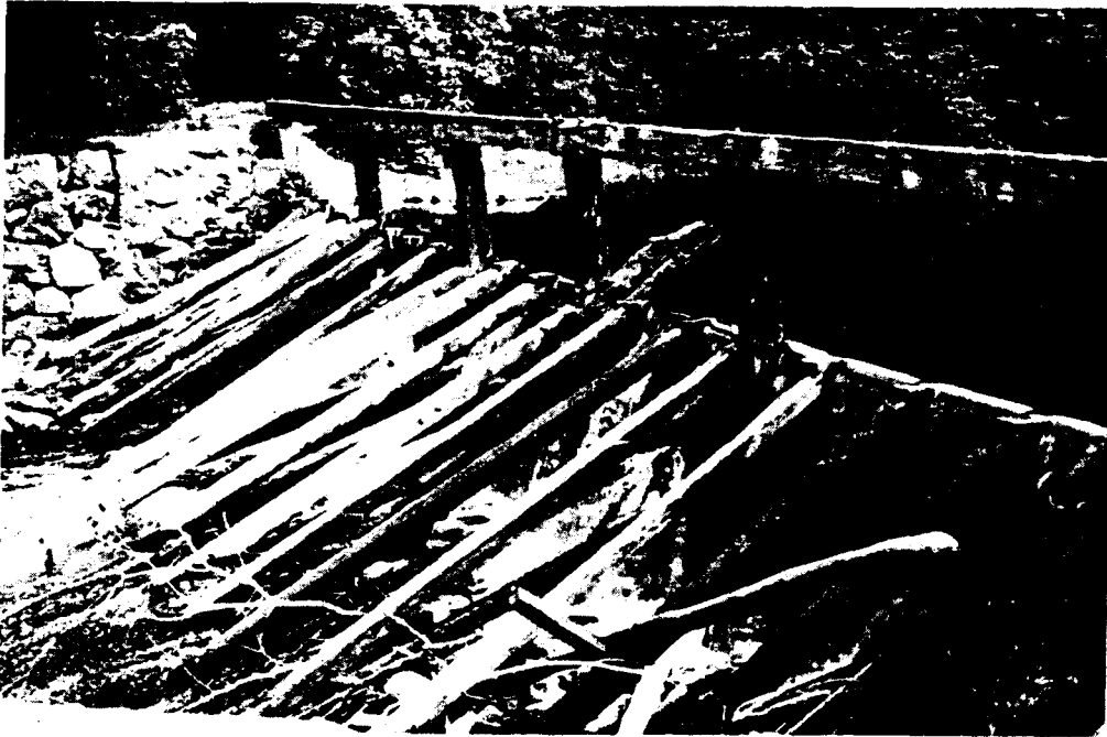
Dam at upper end of East Branch of Westport River at Forge Pond.
