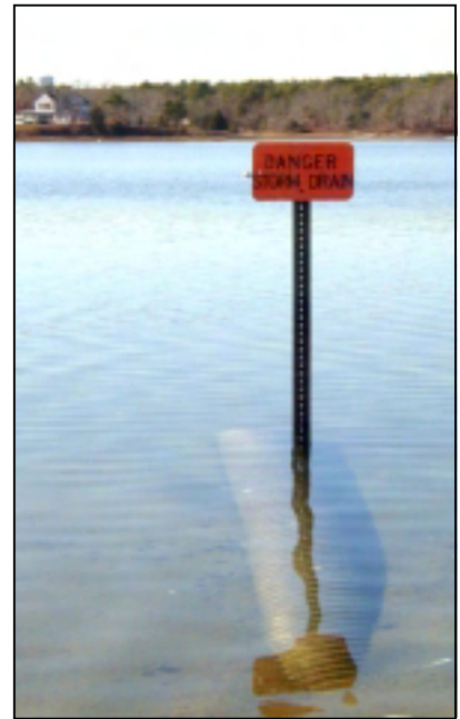
Figure 1. A submerged stormdrain in Wareham.
