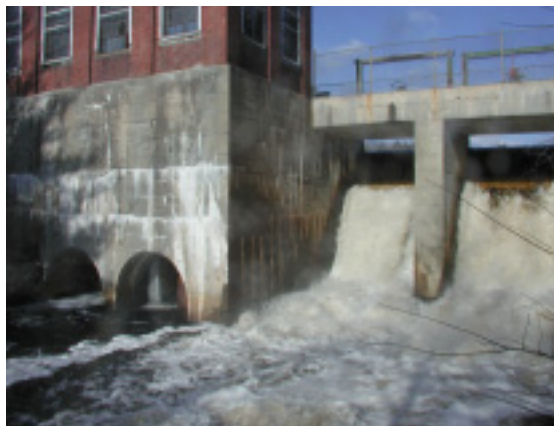
Tremont Mill Pond Dam
